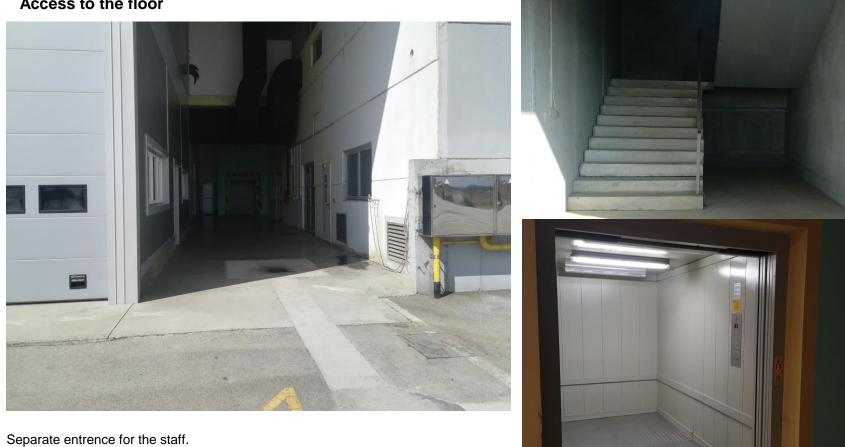
Cargo elevator, with a total load capacity of 4 tons.
